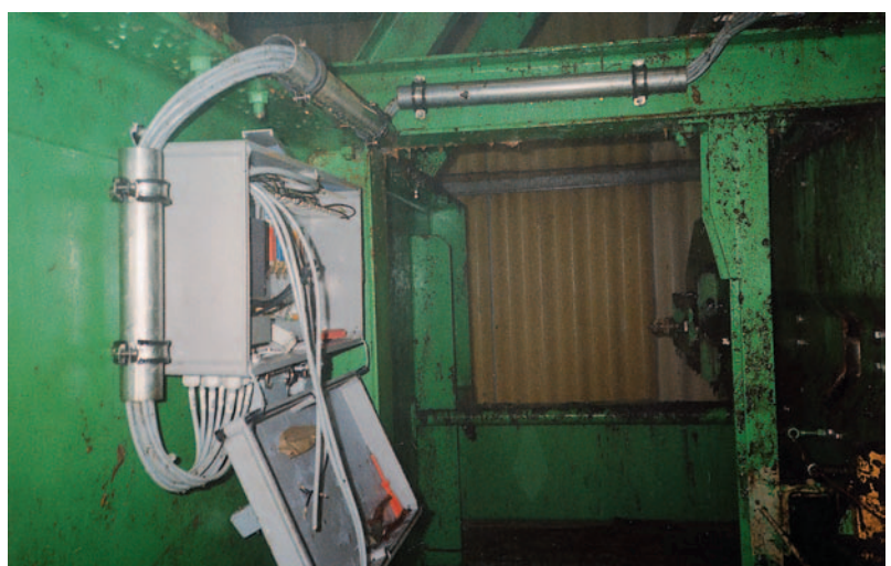
Cable installation in composting work
